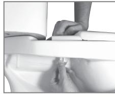
Add washers and nuts to the bolts from underneath the pan. Tighten toilet seat nuts until secure.
