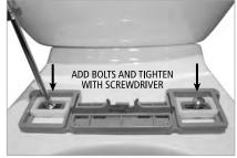
4. Place the frame with the metal washers over the pan holes. If top fixing, fasten the bolts to the rubber nuts using a screwdriver. If bottom fixing, attach the white washers and nuts to the bolts via the underside of the pan holes.
